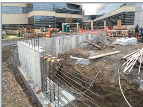
SCREEN WALL FOUNDATIONS
